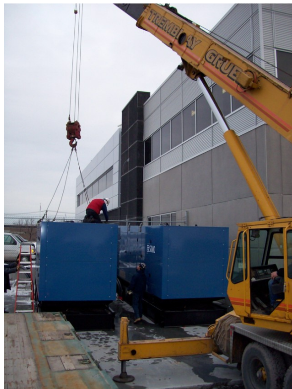
Make: SDMO Model: X910UCTD IV Capacity: 910 kW Engine: MTU 16V2000 Alternator: Leroy Somers Controller: Kerys
